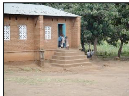
Doorsteps to a classroom
