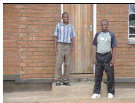
Mr Chintali and Mr Banda, the occupant of the new teacher's house
